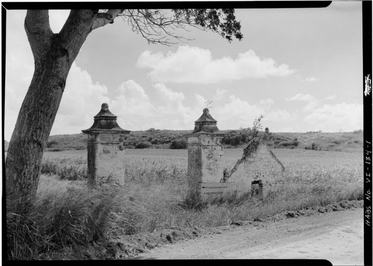
Gateway ruins on Centerline Road near Frederiksted circa early 1930s (Photo by Jack Boucher from the Library of Congress archive)
